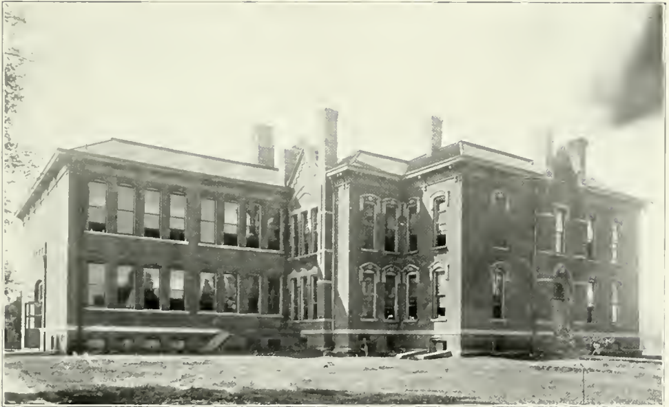
HIGH SCHOOL BUILDING, AMES
